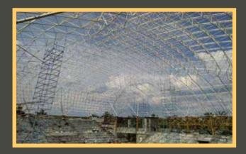
Metal Space Frame is a prefabricated three dimensional space frame system. There will not be a need for any additional work at the site including paint touch up. It is being packed in a special way to protect the powder coated components from scratches during handling at site.
